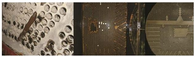
2. The image of the condenser tubes on the left was taken before installation of the Flow-Tech treatment system. The center and right-side images show a dramatic decrease in fouling after the Flow-Tech system was operated. Courtesy: Flow-Tech Systems
